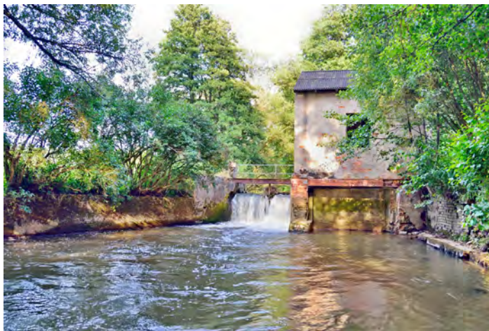
Wehr in Rauhenstein
